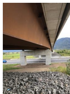
Fig. 2. Weathering Steel patina on Berry to Bomaderry Bridge in NSW.
