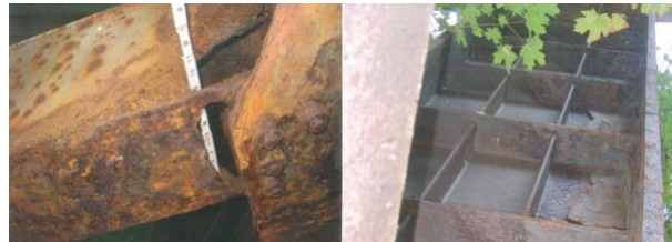
Fig. 6. Corroded elements of Fern Hollow Bridge.
