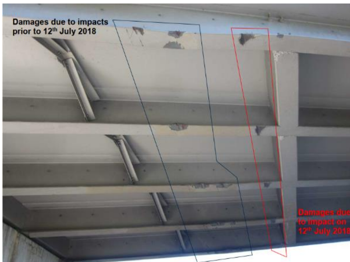
Figure 4: Damage to steel girders above northbound lane – as viewed from the road
