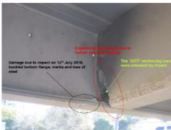
(c) Damaged reinforced concrete cross girder
