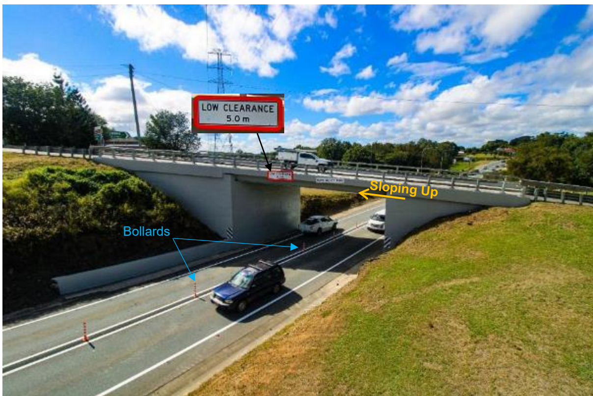
(b) Bollards and new signage indicating vertical clearance
