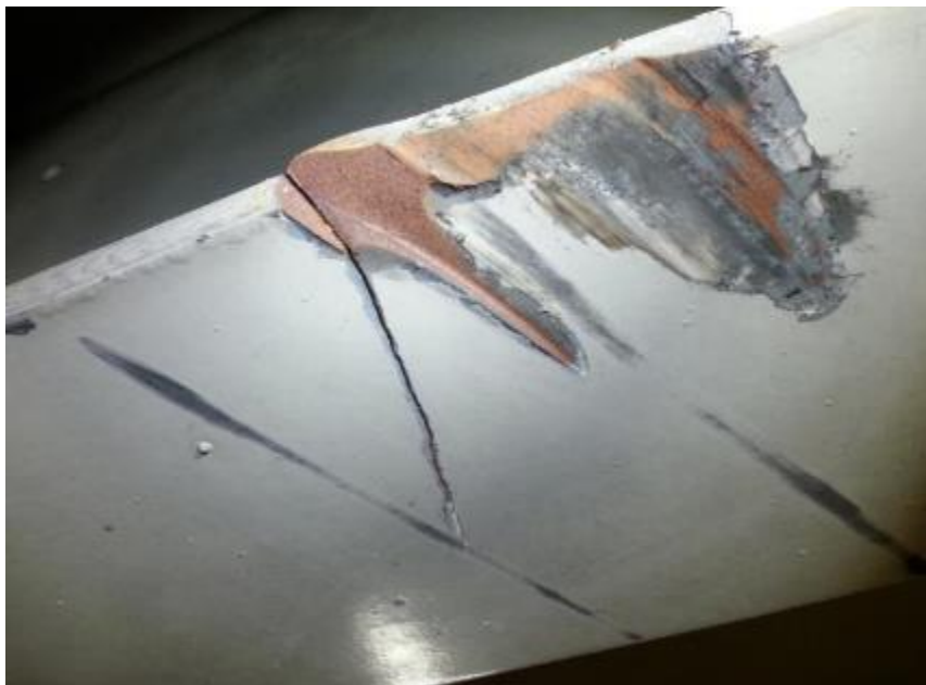
Figure 5: A closer look at the damage to the bottom flange doubler plate of the girders. Cracking and shearing of metal can be seen
