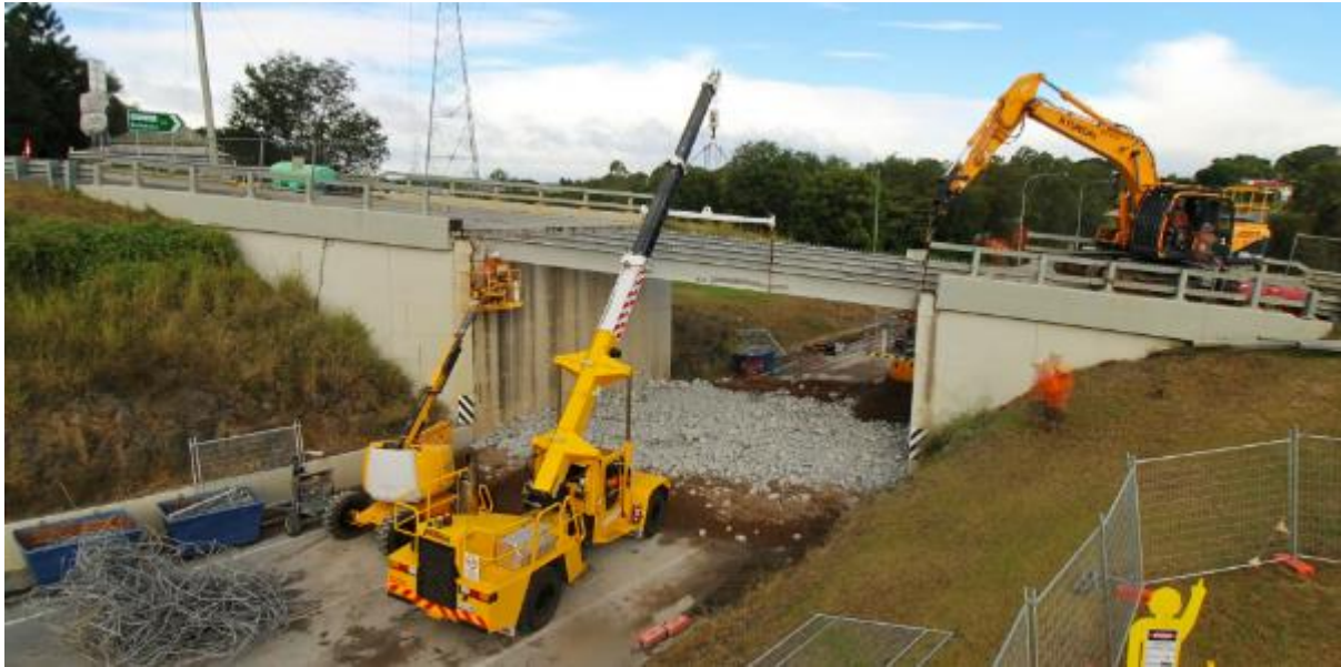
(b) Damaged steel girder removal
