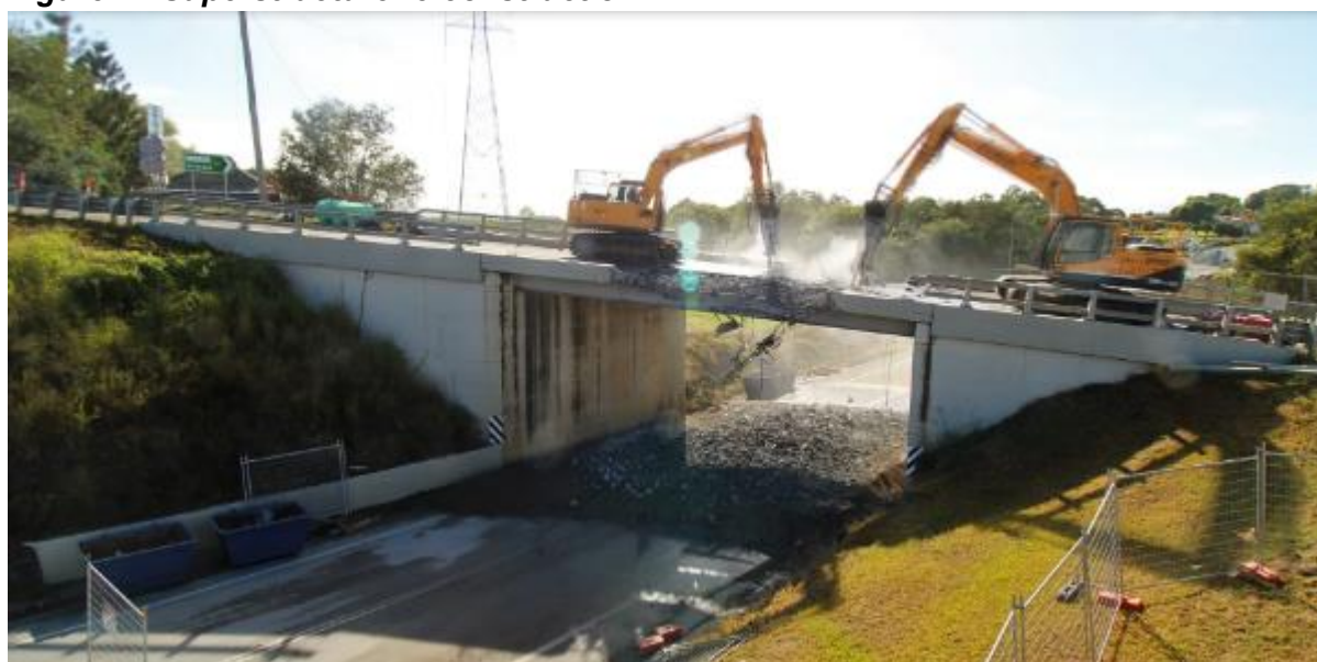
(a) Bridge concrete deck/slab demolition
