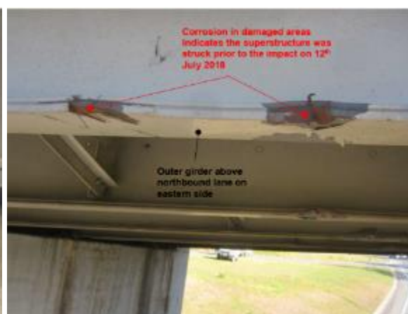
e) Damaged girder due to strike prior to 2018
