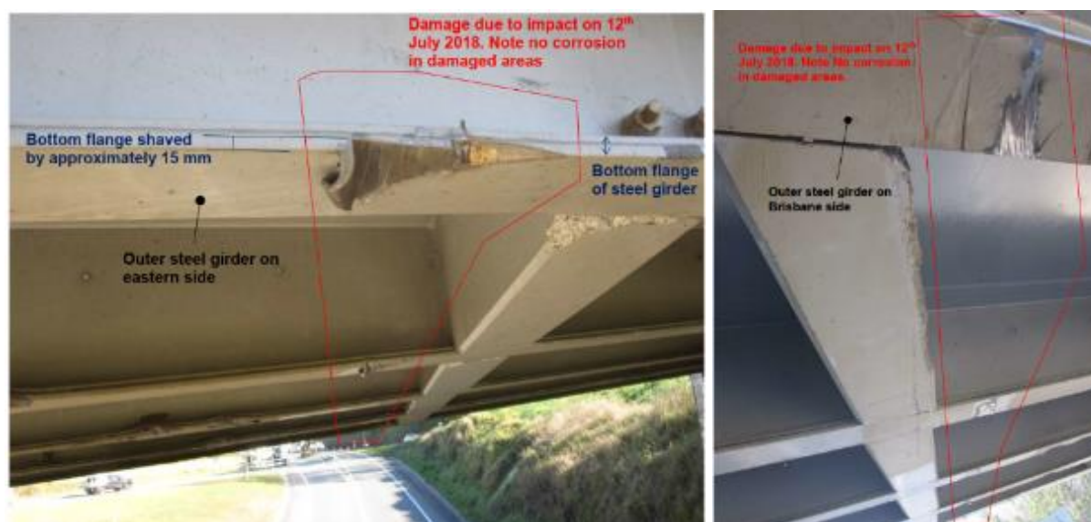
a) Damaged steel girders due to strike in 2018
