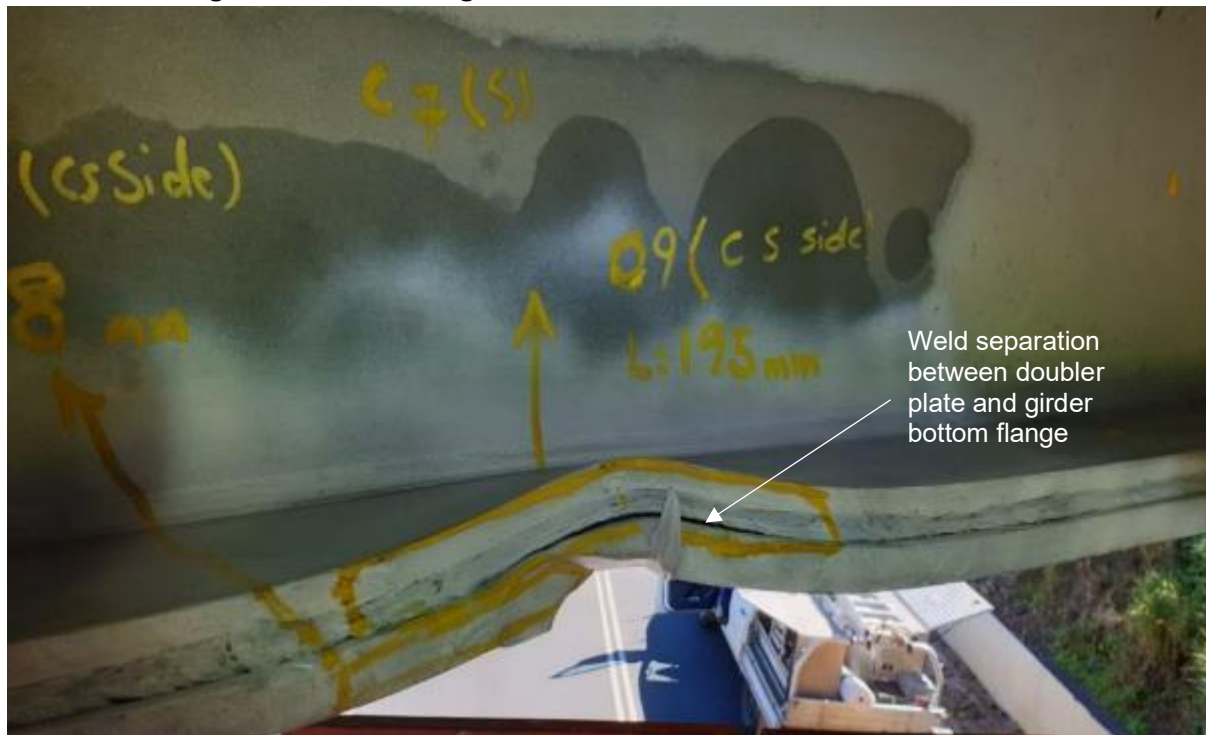
Figure 6 MPI showing weld separation at fillet weld to doubler plate, but no cracks in the 610UB125 girder bottom flanges
