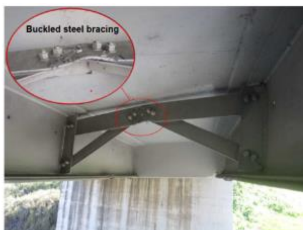
(b) Buckled steel bracing
