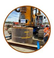
Drilled Shaft Base Cleanliness Evaluation (SQUID)
