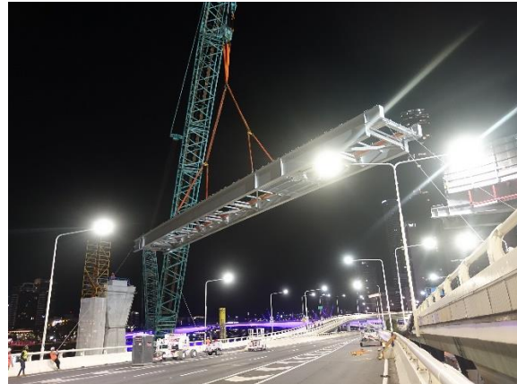
Module 12 Deck Span above the REX
