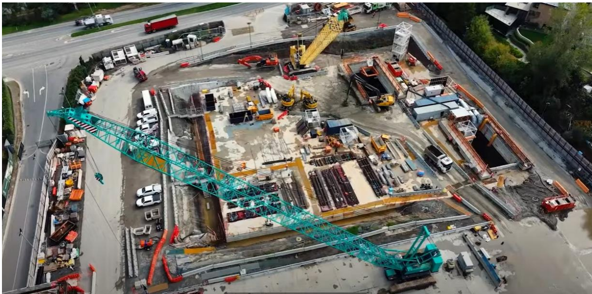
Image 1 – Bulleen Cut and Cover tunnel roof slab at SEM portal (Source: North East Link, Zoning in on SEM tunnelling - YouTube )
