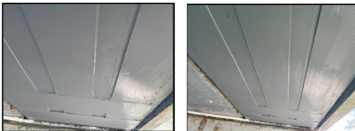
Figure 9 CFRP installed on plank soffit in Heywoods Bridge
