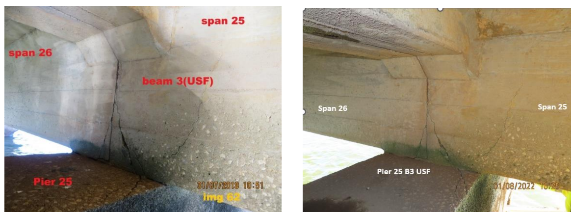
Figure 18 Comparison between photos of L3 inspection 2018 and 2022
