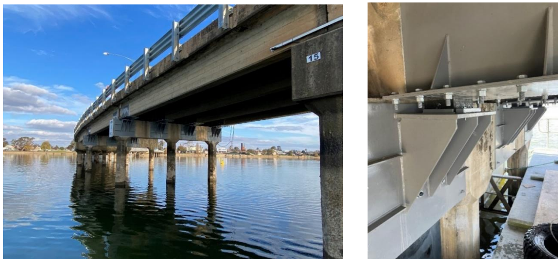
Figure 21 Post installation photos showing steel plate bracket installed
