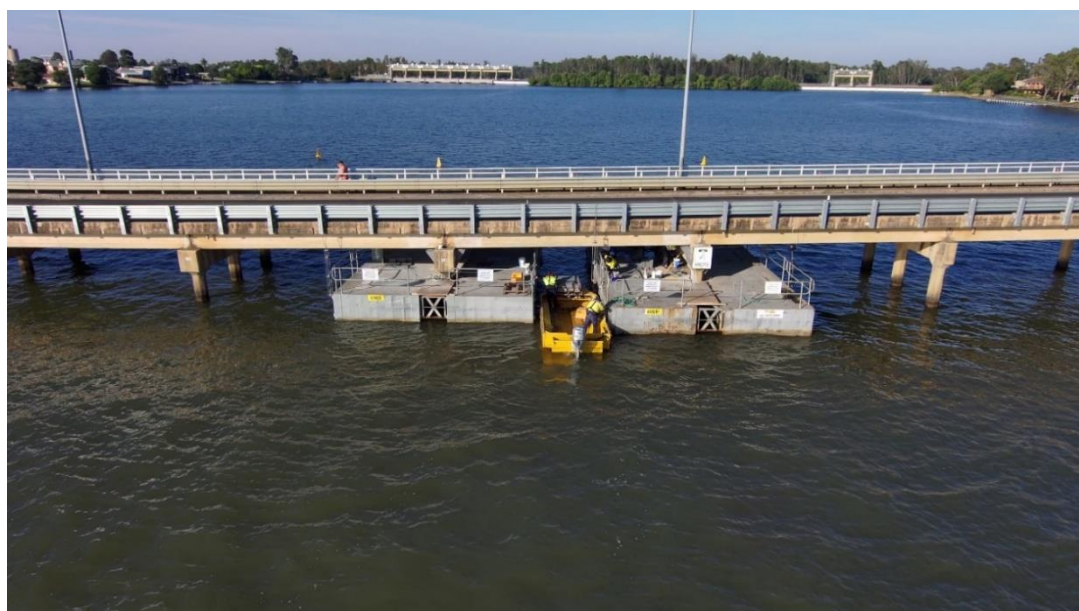
Figure 20 Barge setup for installation of the steel plates
