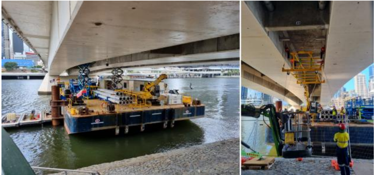
Figure 13 Barge works with lifting frame
