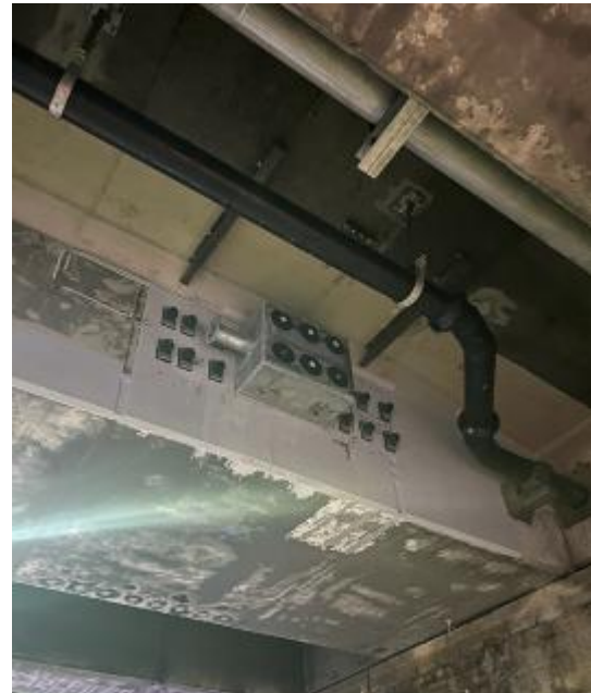
Figure 27 Example of installed blister
