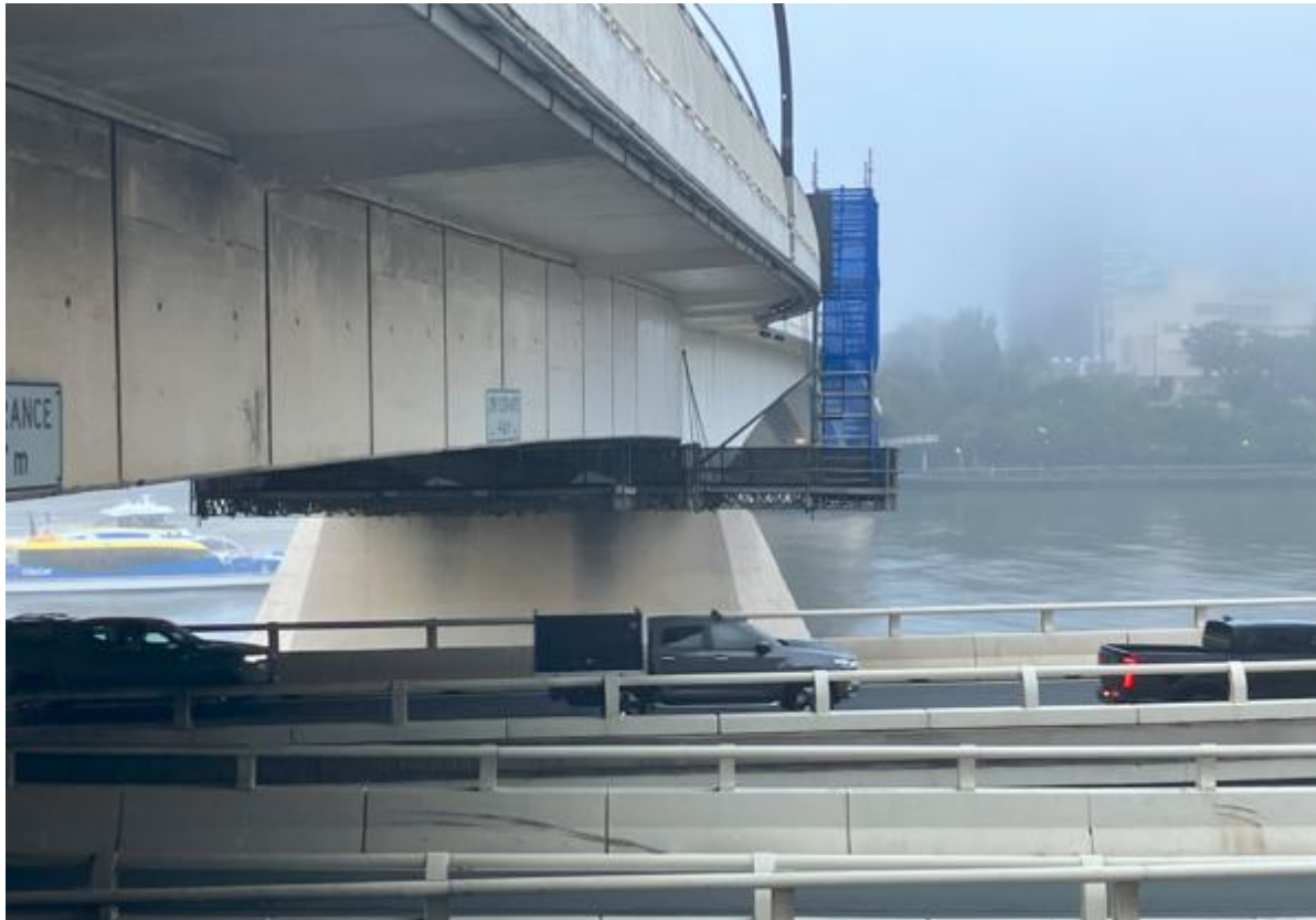
Figure 18 Hanging scaffold at the Brisbane City side with access from above
