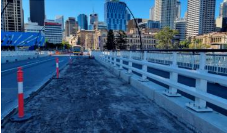
Figure 34 Example of lane configuration when removing asphalt wearing course
