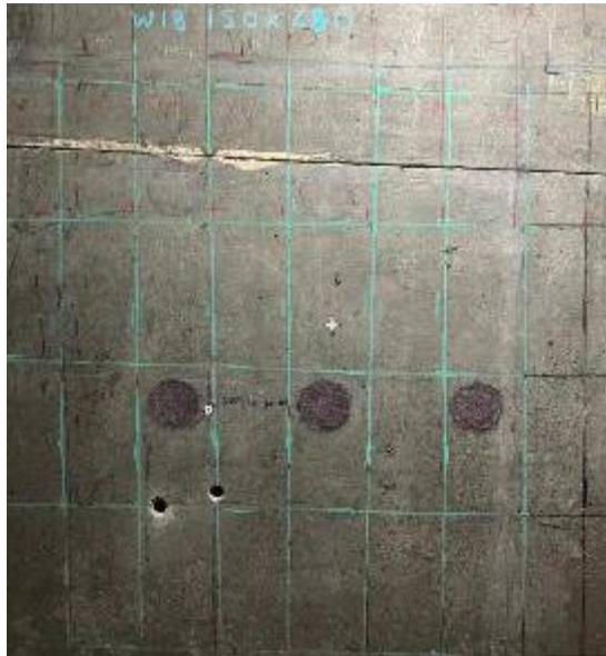
Figure 9 Rebar marking after scanning
