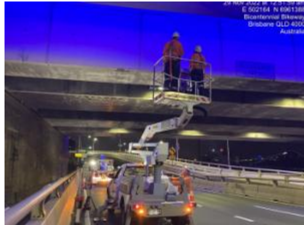
Figure 21 Vehicle mounted EWPs
