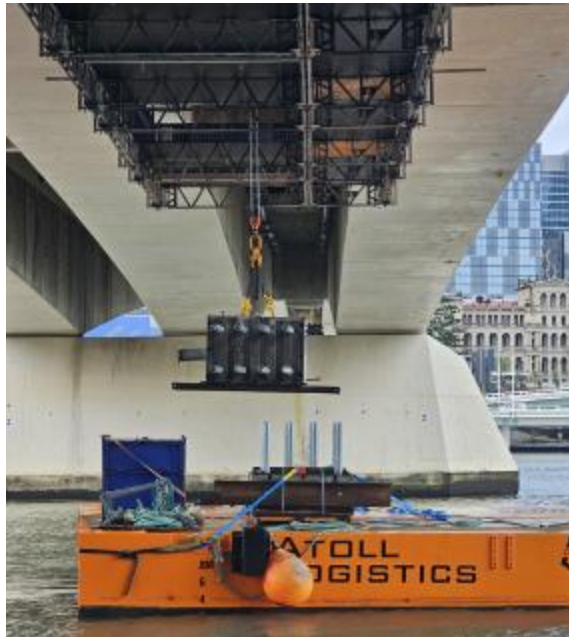
Figure 26 Blister installed from the river
