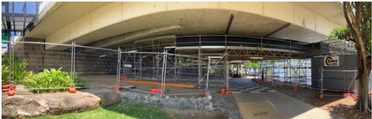
Figure 17 Looking up at hanging scaffold beneath the bridge at the Southbank Precinct side
