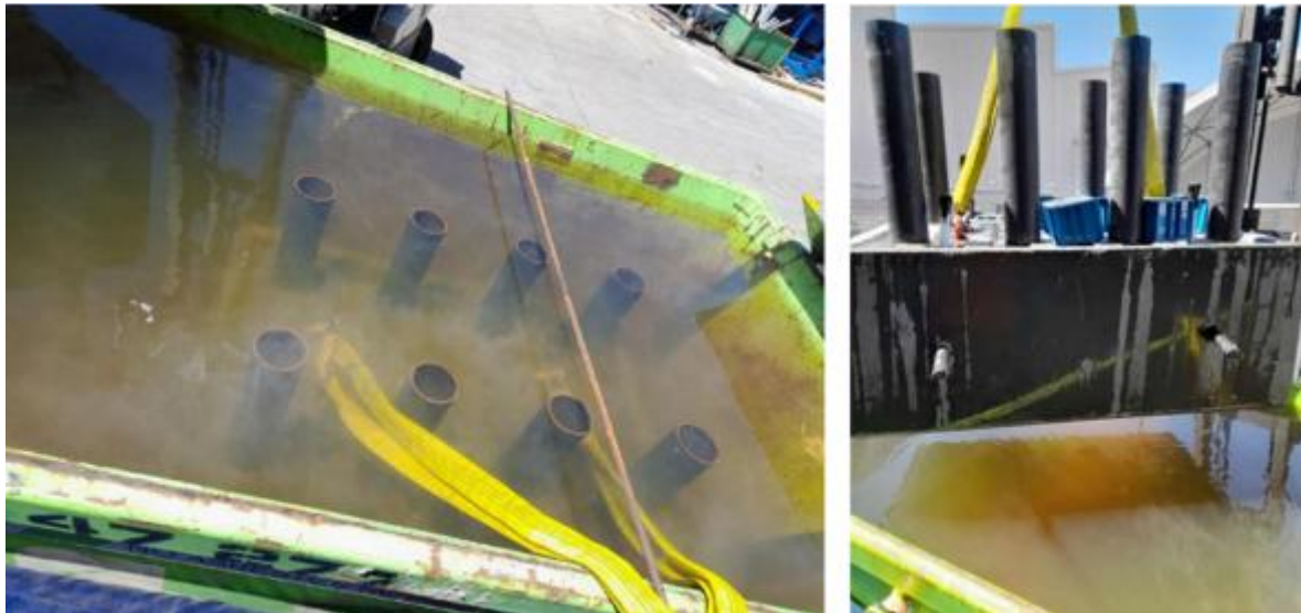
Figure 24 Use of hot water curing baths
