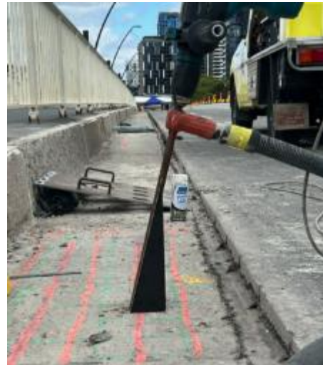
Figure 33 Fabricated templates for bolt groups
