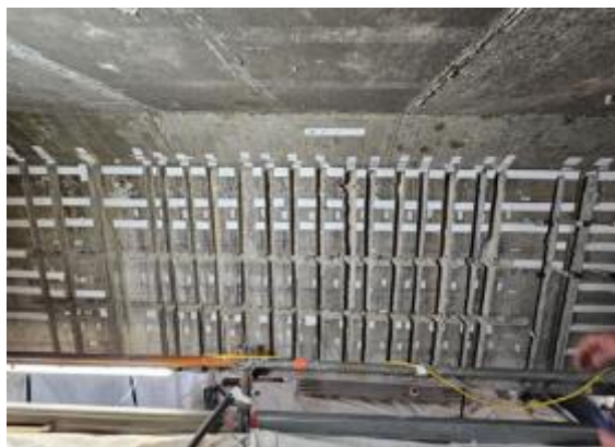
Figure 30 Vertical NSM grooves in web
