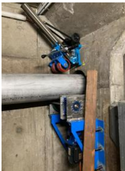
Figure 11 Pipe pushing over the Riverside Expressway
