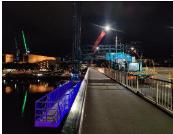
Figure 20 Use of UBIU under lane closure
