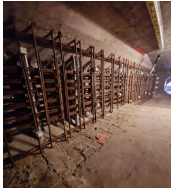
Figure 23 Restricted space working
