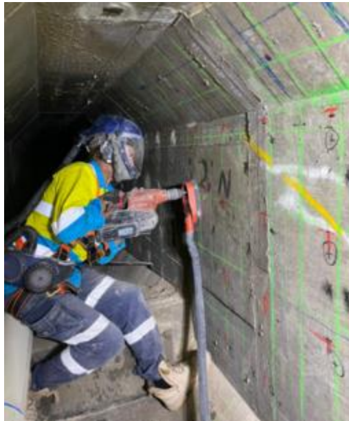
Figure 22 Confined space working
