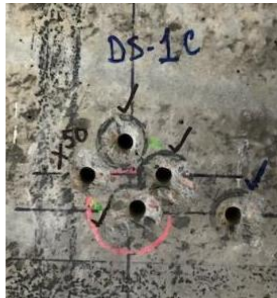
Figure 10 Pilot holes after GPR scanning
