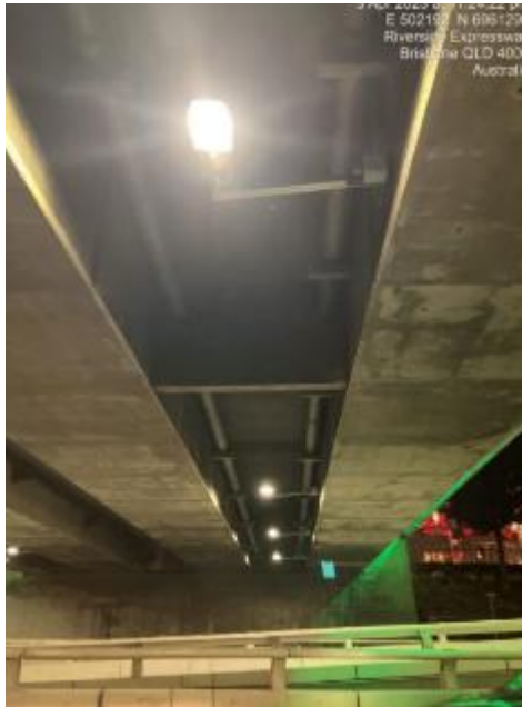
Figure 14 Sewer lines pushed through and over the Riverside Expressway
