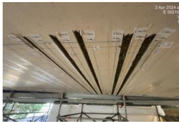
Figure 31 Overhead NSM grooves in soffit
