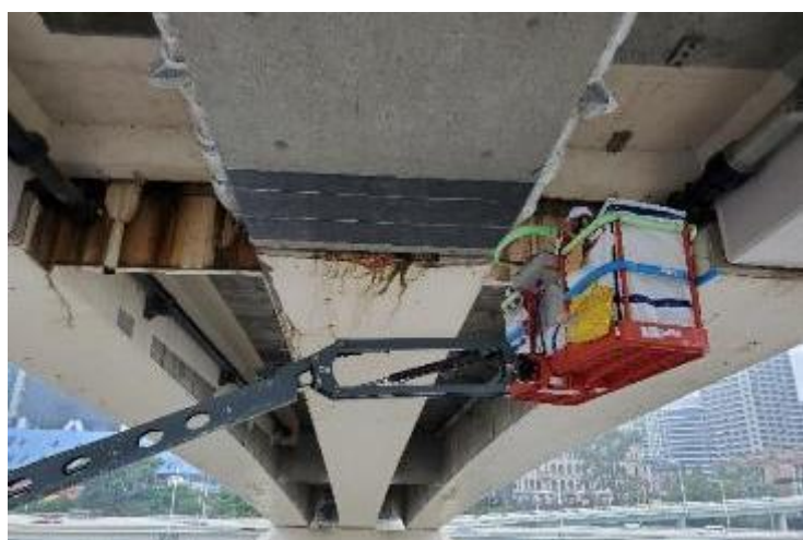
Figure 29 Installation of CFRP at Mid-Span Half Joints
