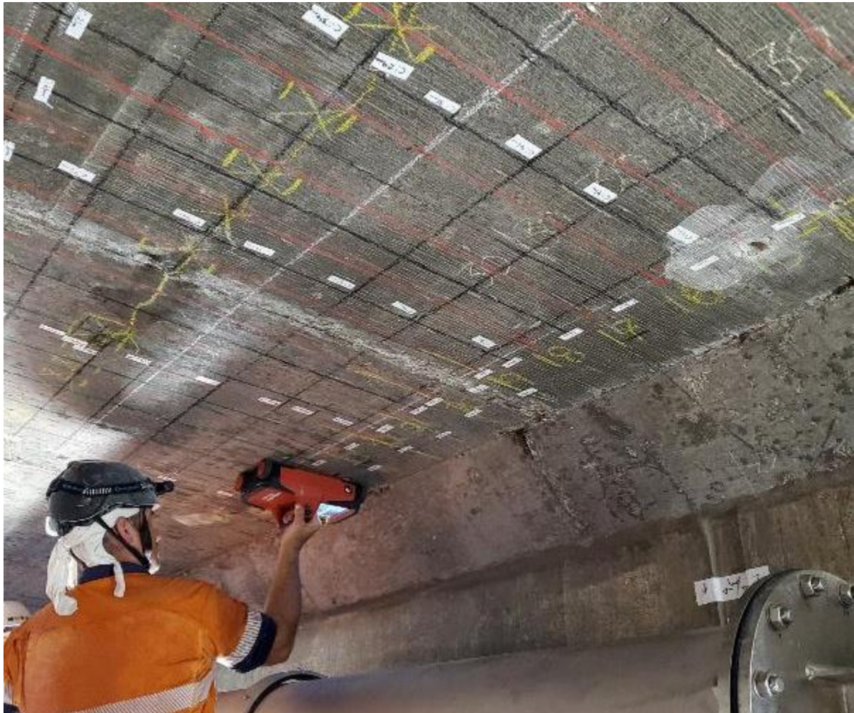
Figure 8 Reinforcement scanning and marking on the bridge soffit
