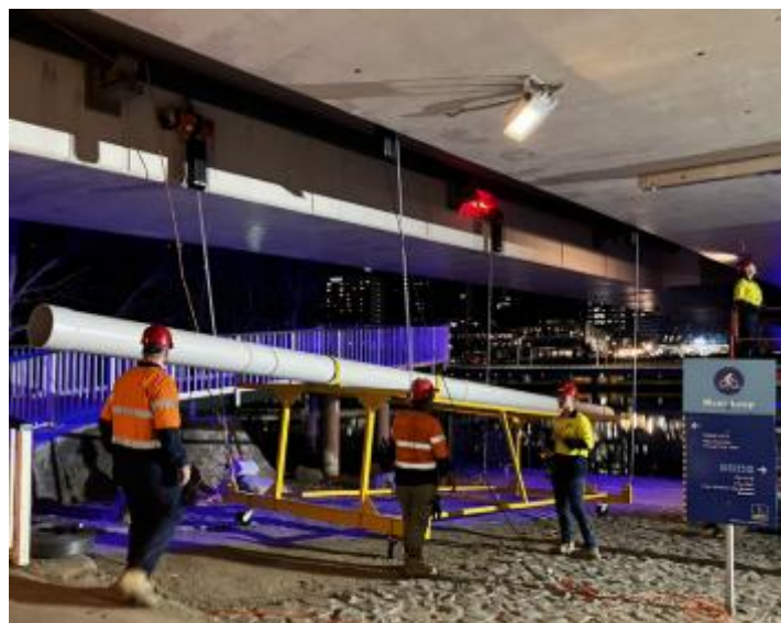
Figure 12 Lifting frame with access from Clem Jones Promenade
