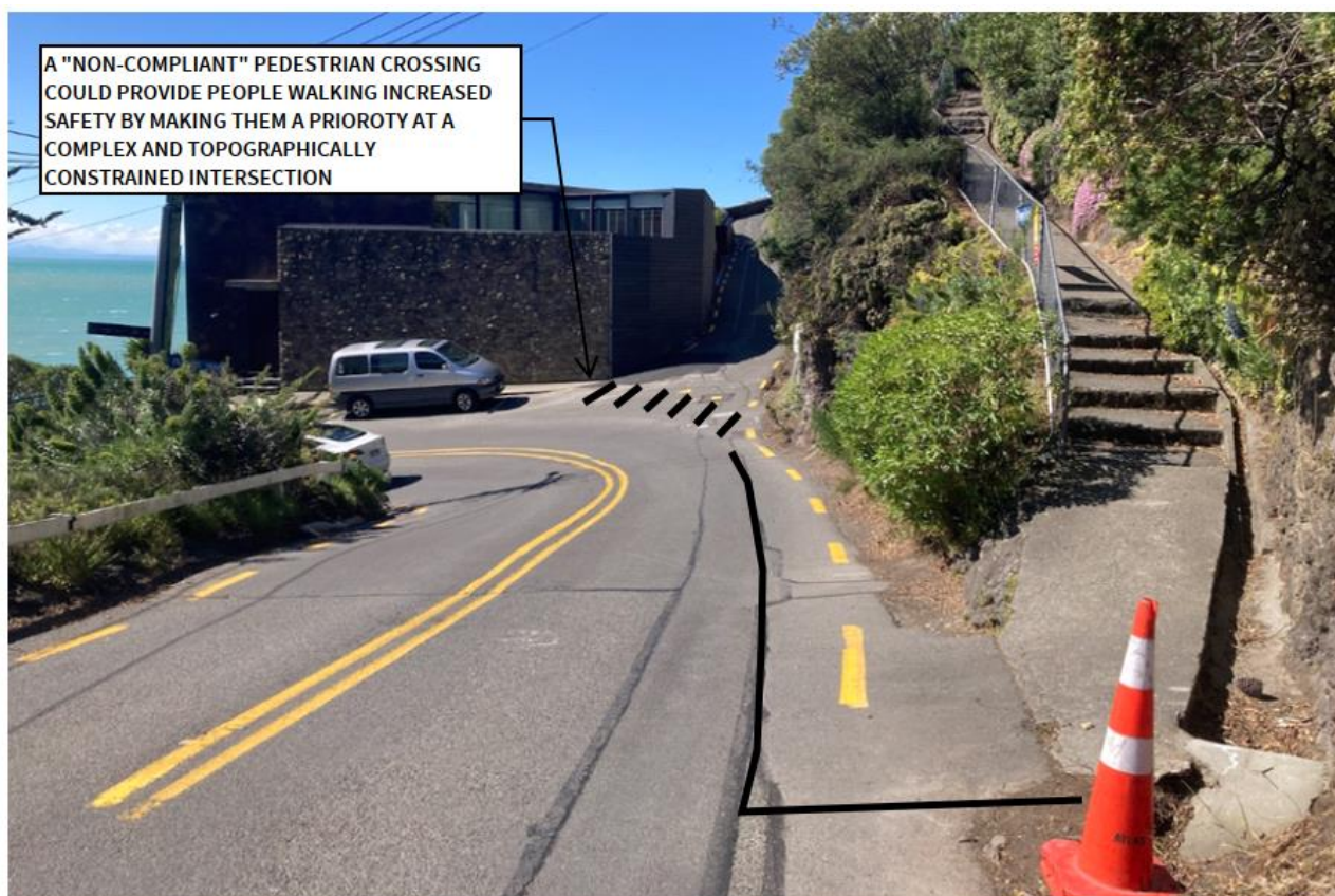
Figure 1. Footpath in Christchurch stops abruptly to due steep topographic constraints. A stepped walkway provides access to houses on the Scarborough hill (Christchurch, 2025)
