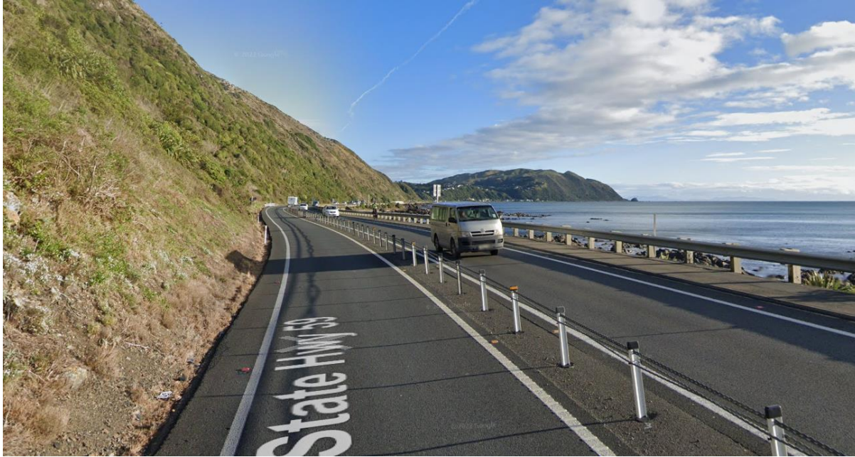
A typical retrofitted corridor
