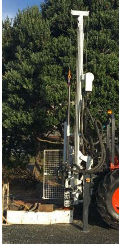
Standard Penetration Test (SPT)
