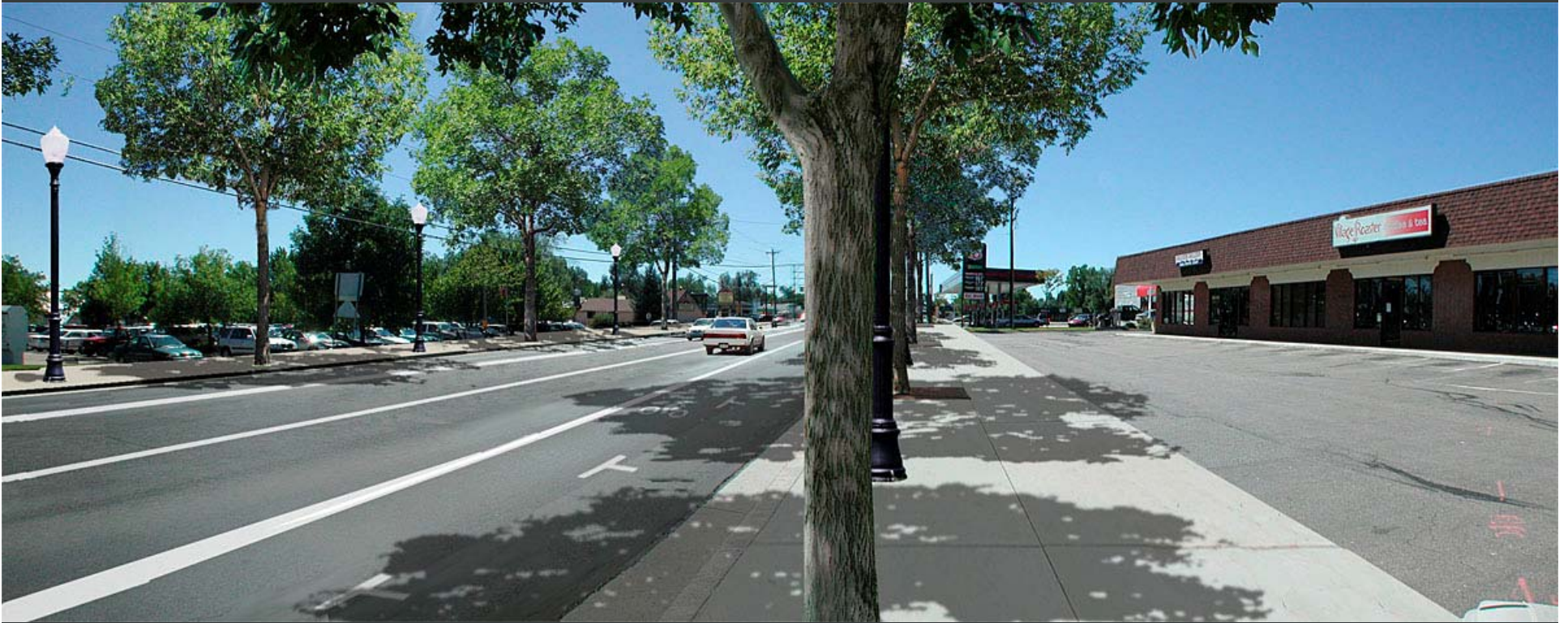
Public street improvements
