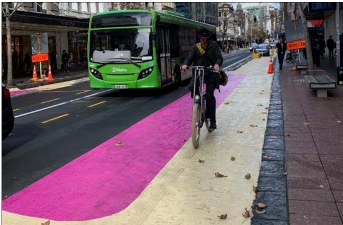
Figure 4: Coloured surfacing to delineate space for people in July 2020
