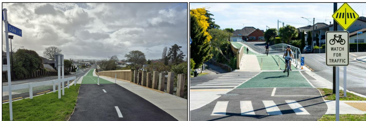
Figure 10: Constructed Boardwalk (Western End – Left, Eastern End – Right)
