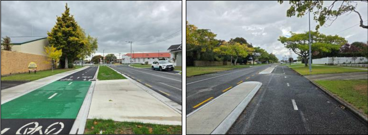
Figure 6: Berm Buffer on Bryce St (Left) and Concrete Median Separators on Alpha St (Right)
