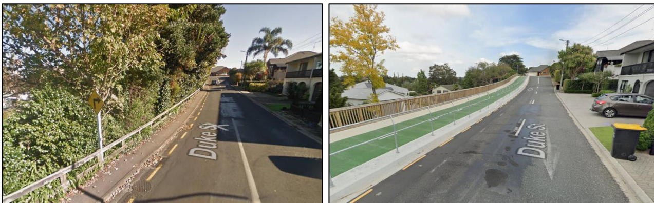
Figure 12: Duke St Before (Left) and After (Right)
