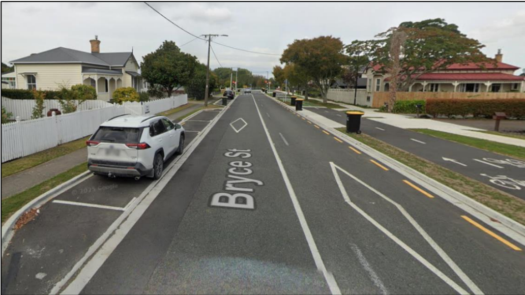
Figure 8: Recessed Parking Bays on Bryce St (20 m wide Road Reserve)
