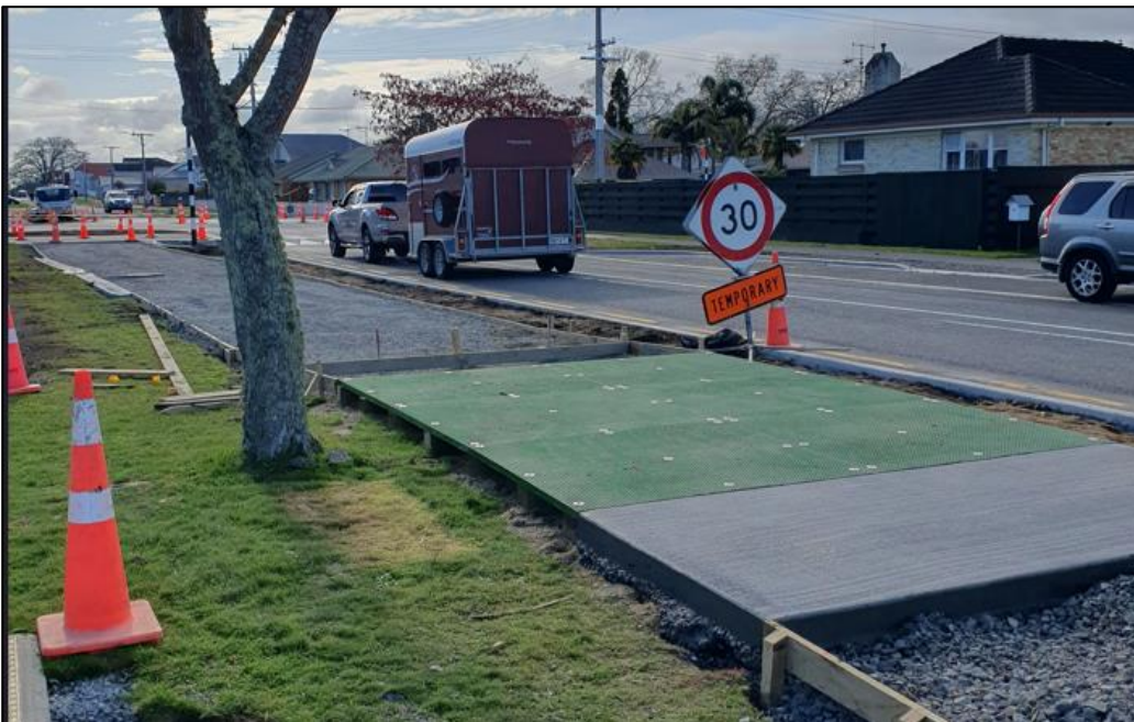
Figure 9: Installation of FRP Panels
