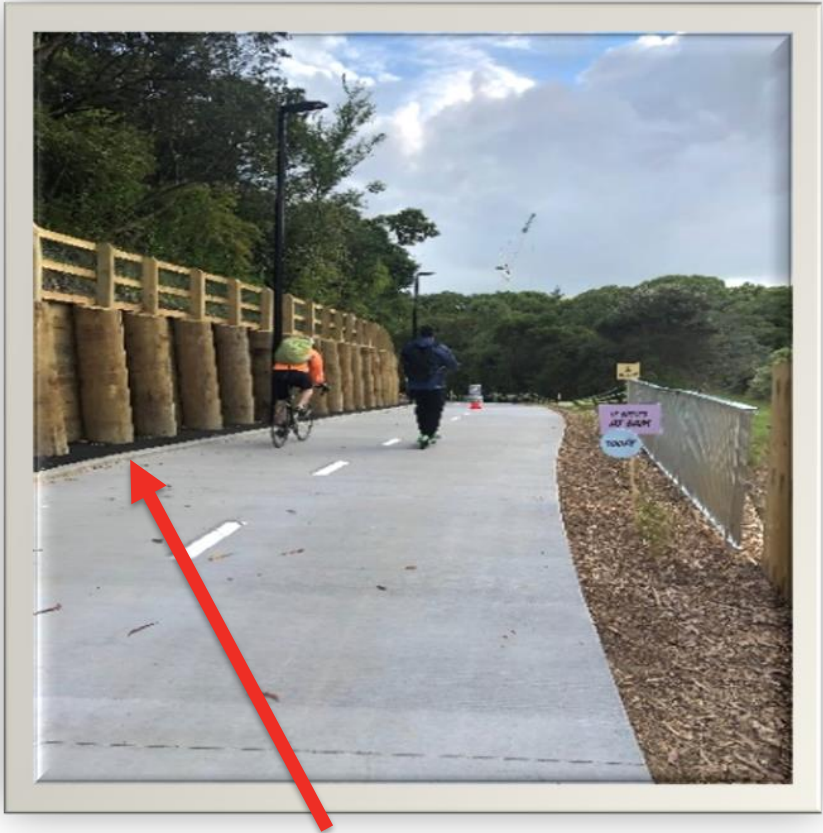
Kerb edging to retaining wall
