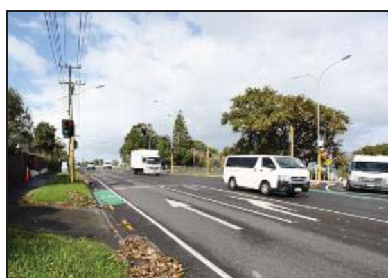
Figure 4: Downhill vehicles northbound on Carrington Rd
