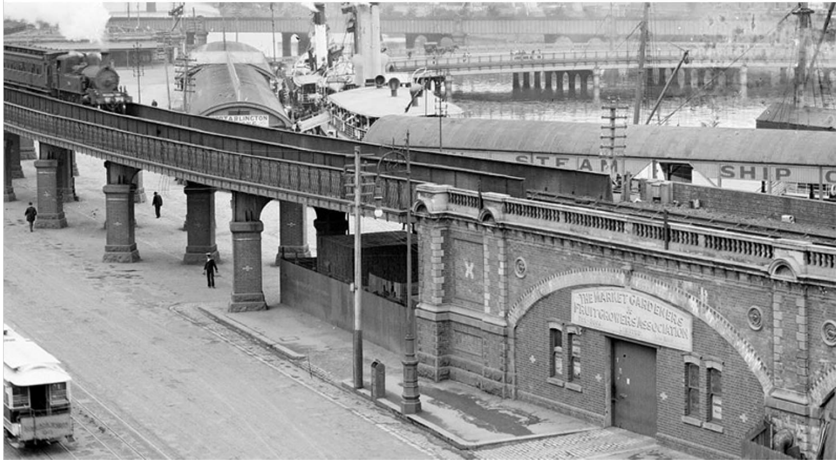
Flinders Street viaduct, circa 1910. Source: Museum of Victoria
