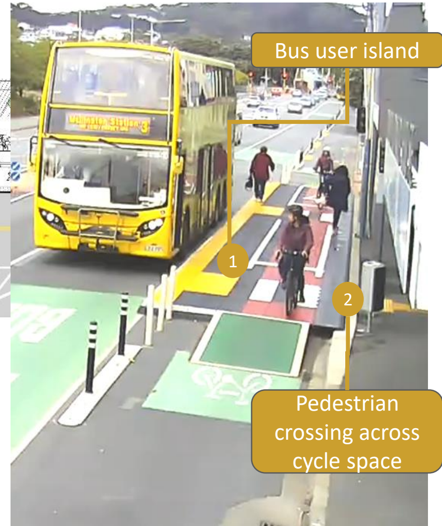
Bus bypass design, Wellington (followed Waka Kotahi Bus Design Guide)
