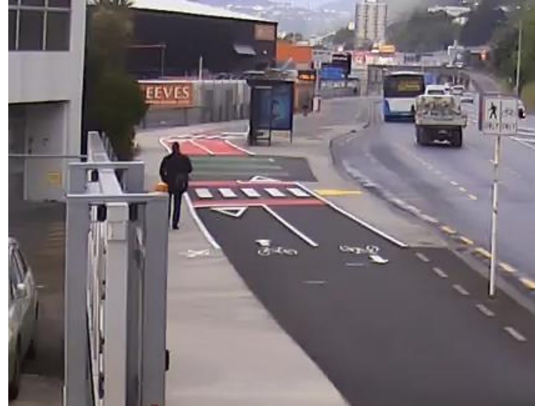
Shortest, straight crossing angle (with markings)
