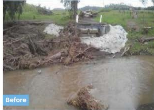
Villis Bridge Scenic Rim Regional Council
