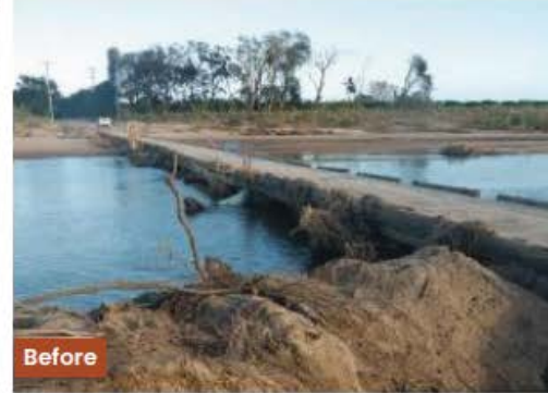
Inverdon Bridge Whitsunday Regional Council
