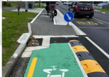
Figure 19: Example of catch pits at raised safety platform
