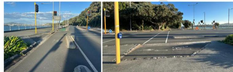
Figure 24: Jug handles provide waiting space for cyclist turning right on T-Intersection of Tamaki Dr and Ngapipi Rd
