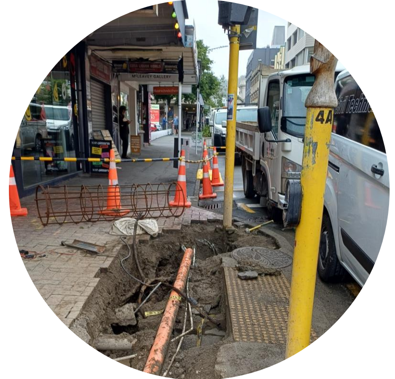
Signal upgrades Utility Maintenance
