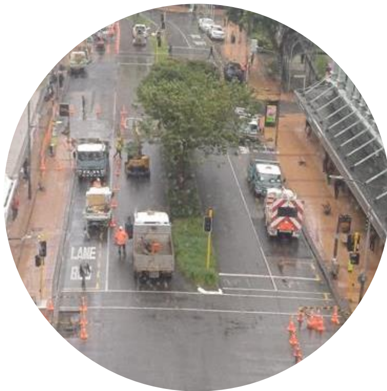
Dig outs Resurfacing Utility Maintenance
