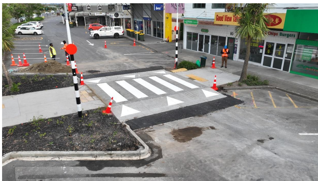
Figure 2: Overnight installation of Pre-cast concrete RSP (Photo: Fulton Hogan, 2023)
