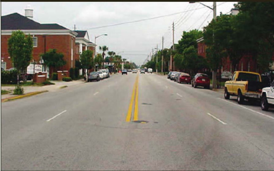
Figure 1. Photo. Four-lane configuration before road diet.
