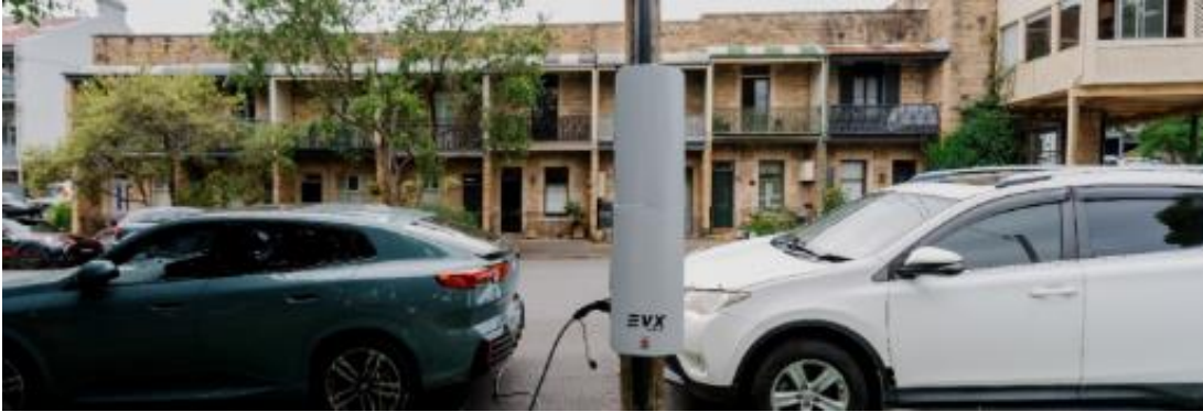
Figure 5 Pole mounted EV charging
