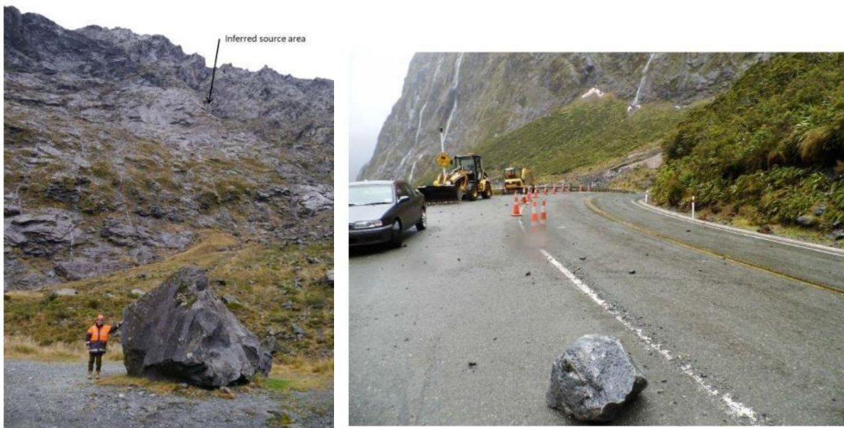
Figure 2. Rockfall at Homer Tunnel (Supplied)
