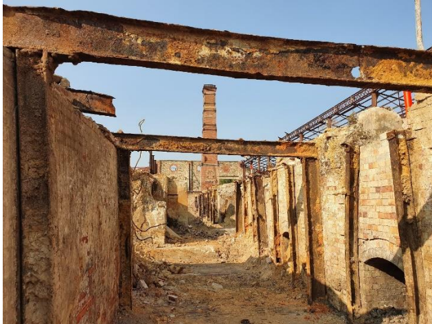
Retort House No.4 – Horizontal underground retorts re-discovered in 2019
