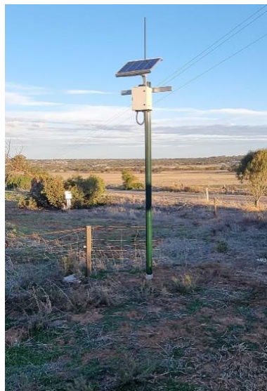
Figure 4: Portal in situ
