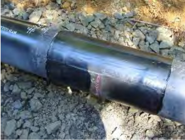
Anti-corrosion coating installation. Surface Preparation Holiday Test
