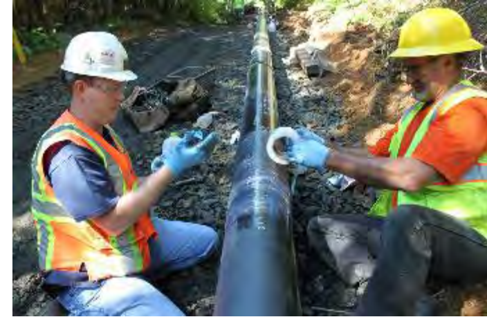
Compression Film Installation Two Passes, 50% Overlap
