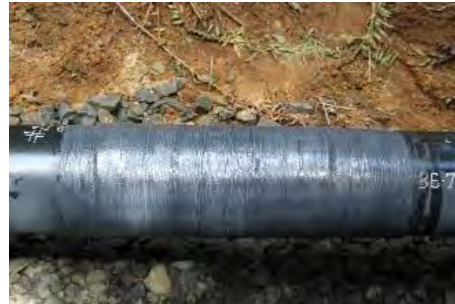
Composite is ready to pull when Shore D is > 60
