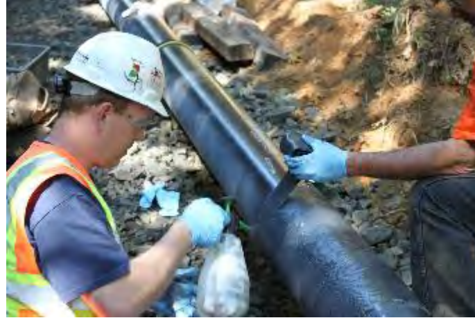
Composite Installation Single Pass, 50% Overlap Water Activation
